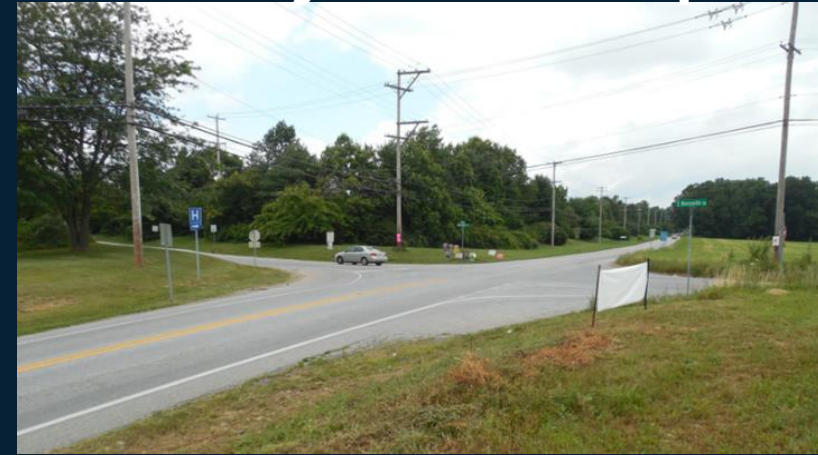
Manor Rd & Reeceville Rd Roundabout
